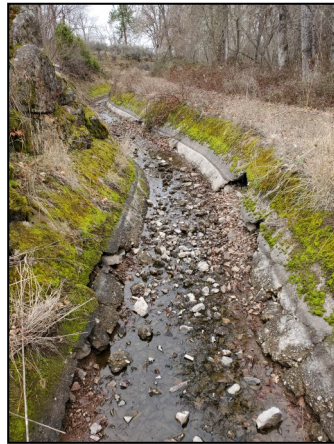
Joint System Canal
