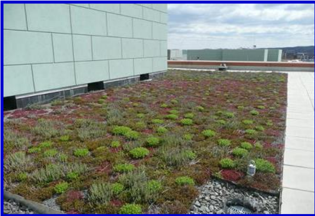
Extensive Green Roof in Washington D.C. Source: US EPA
